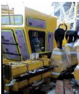
5. Cabs, trolleys and hooks were staged on the floor of the new bay.
