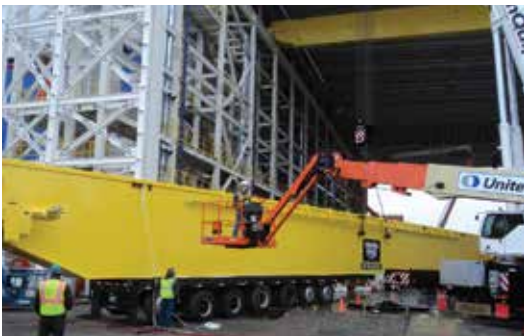
7. The second girder of the East Crane.
