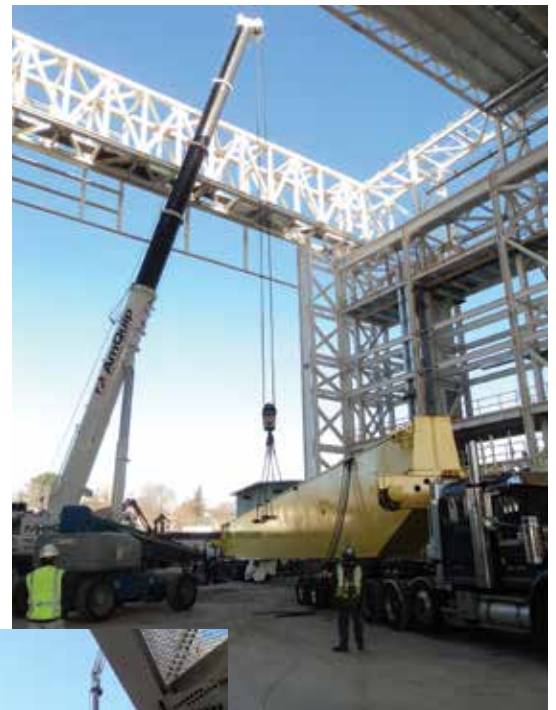
5. Cabs, trolleys and hooks were staged on the floor of the new bay.
